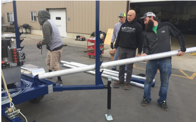
Figure 6. Insert Lower Section of Aluminum Pole
