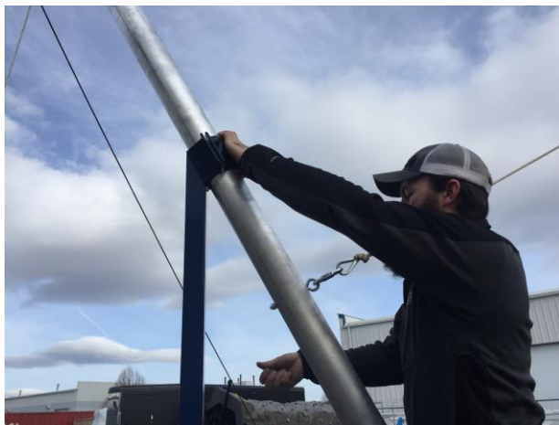
Figure 27. Putting the Pole Into Place and Clamping
