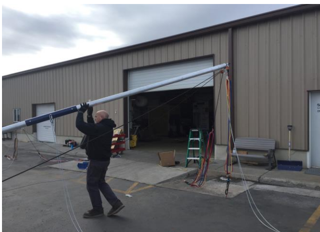
Figure 29. Lifting the Pole by Hand
