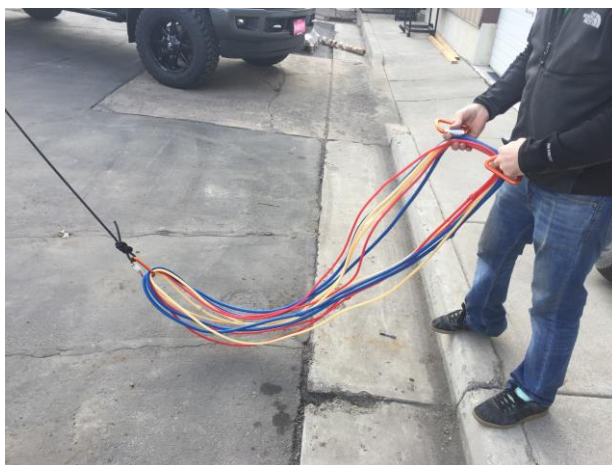
Figure 18. Attach Bungees to the Tension Rope
