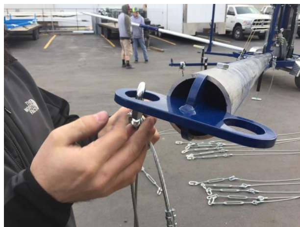
Figure 12. Attach Long Guy-Cables to the Top of the Pole
