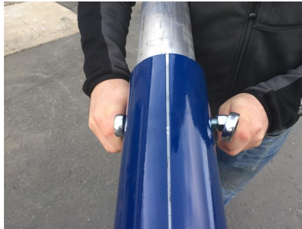
Figure 10. Tighten Bolts to Secure Upper Section
