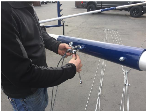
Figure 11. Attach Short Guy-Cables to Middle Section
