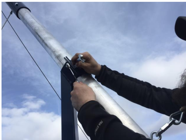
Figure 28. Tighten the Bolts to Secure the Pole.
